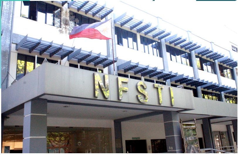
The 3-Storey NFSTI Building which envisions to be The Center of Digital Forensic Training and Education as well as to be the Center of Continuing Professional Training and Education in Crime Investigation and Forensic Science
